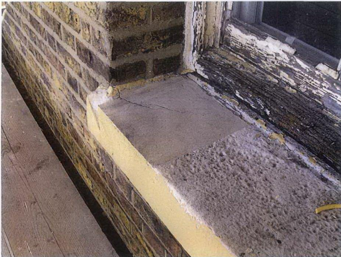
Photo 7: Sill of window 313/W1e showing from where stone sample was taken.
