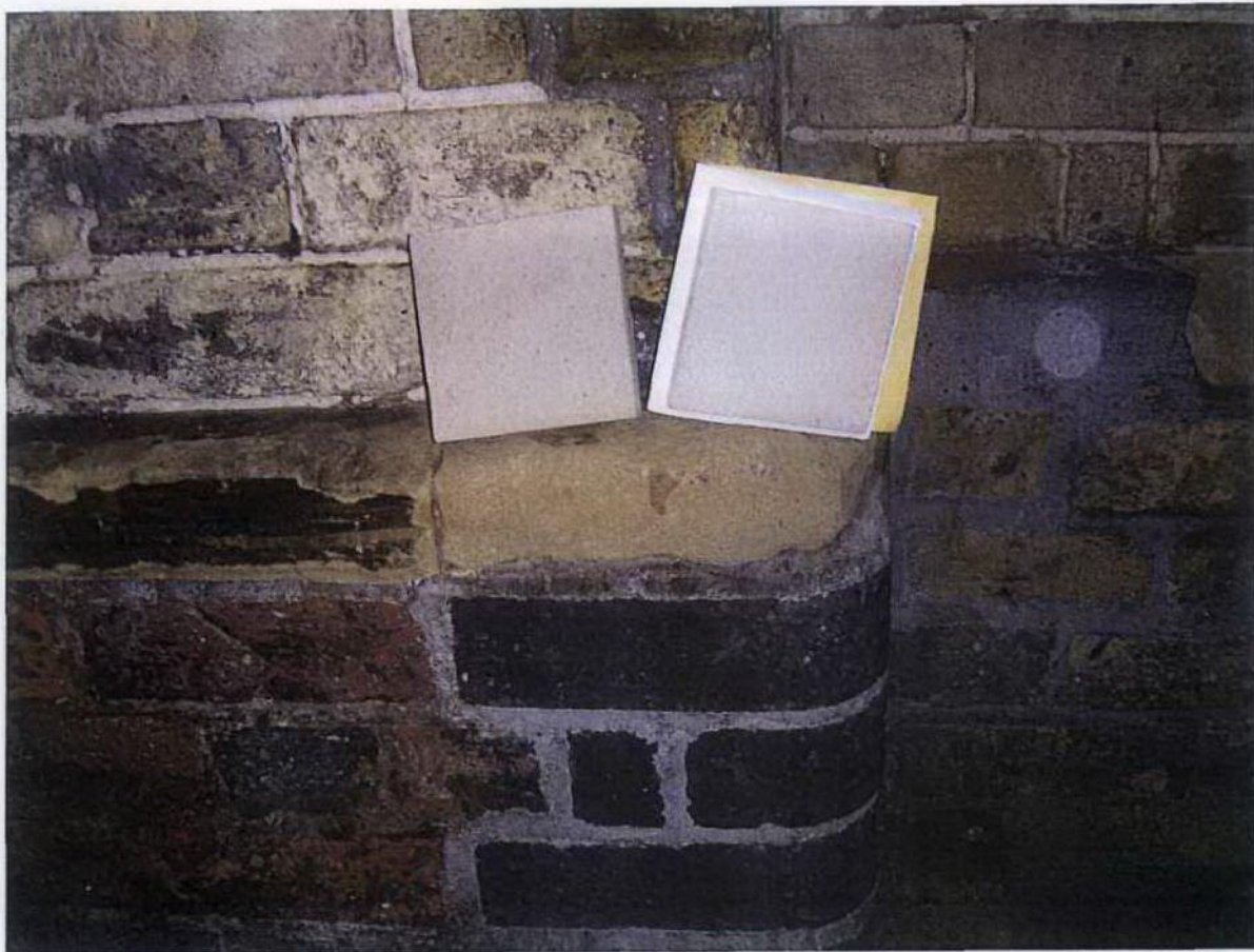
Photo 1: Existing plinth with a sample of Dunhouse Blaxter on the left and Witton Fell Fine Grit on the right. It has been agreed that Dunhouse Blaxter is the best match.
