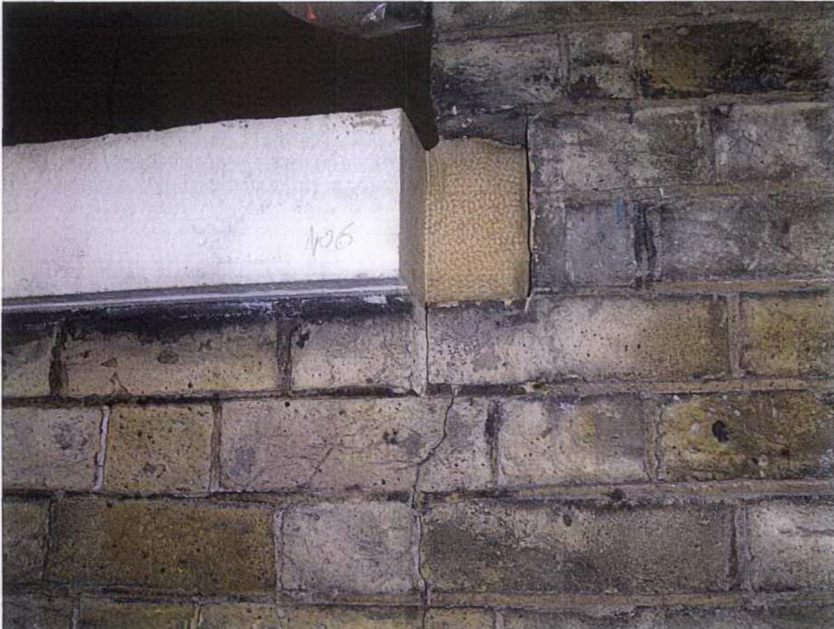
Photo 3: Painted sill of window 108/W2e showing cut out ready for an indent repair.
