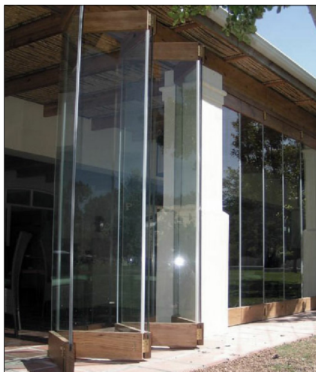
Folding frameless door in 4 sections to both extensions to allow full opening of aperture
