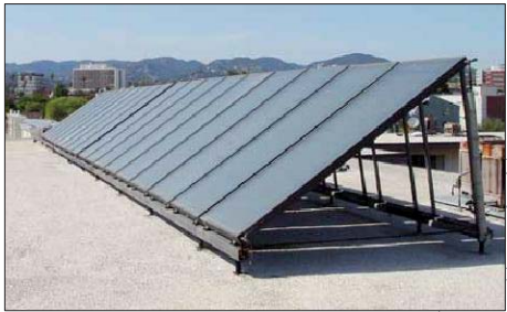
AREA 20m² OF SOLAR PANELS FOR HOT WATER GENERATION. TO BE ANGLED AT 30-40° TO THE PERPENDICULAR AND CIRCA 1-1.5m AT THEIR HIGHEST POINT - PANELS TO BE SOUTH FACING
