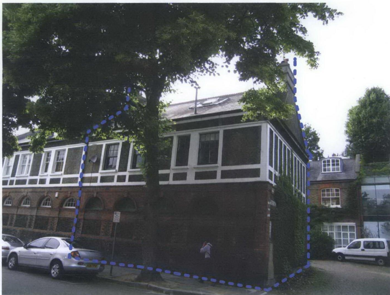
02. Existing rear elevation of No 8 Belsize Court Garages (view from Belsize Lane)
