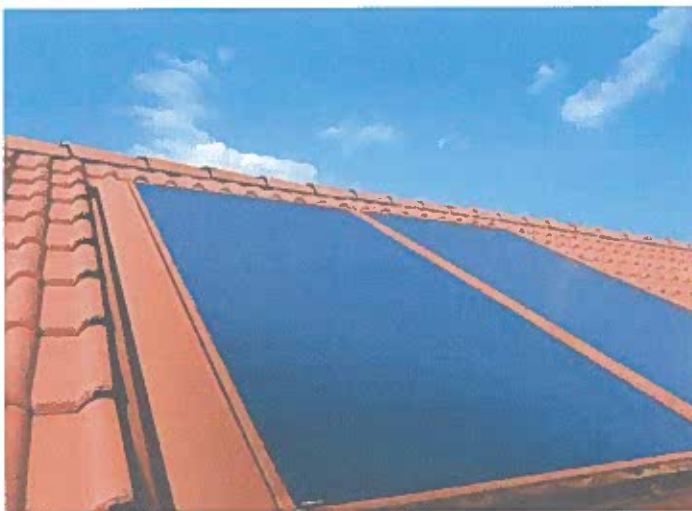
Figure 4: Flat Plate Solar Thermal Collector (© http://www.inbalance-energy.co.uk )
