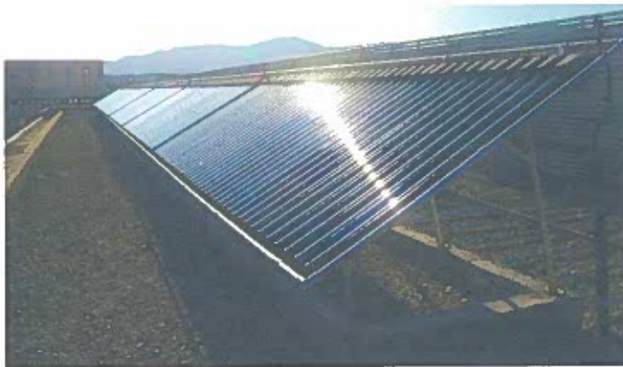
Figure 3: Evacuated Tube Solar Thermal Collectors (Creative Commons License)
