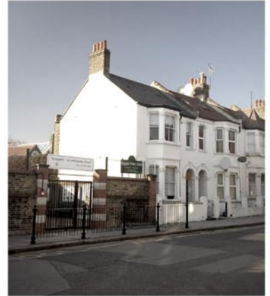
FIG.1 View of the front of the property and neighbouring school / houses.
