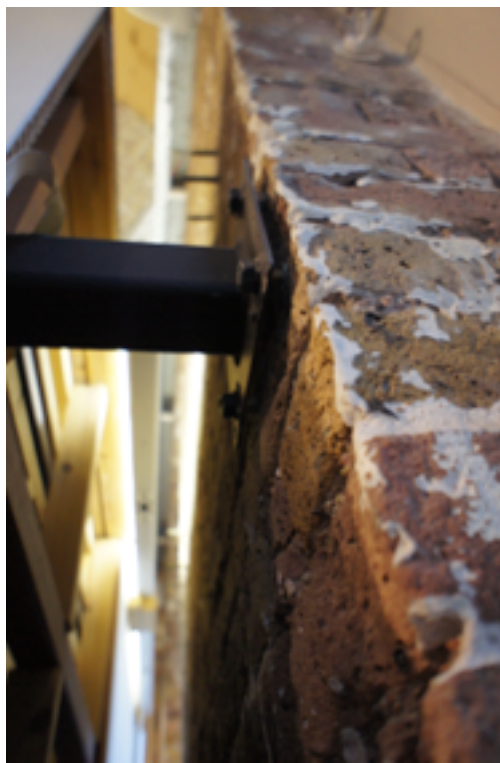
Typical fixing detail of first floor fixtures to existing brickwork
