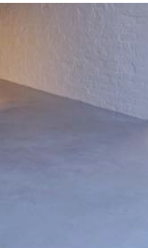
power-floated concrete floor with colour hardener white-painted exposed brickwork
