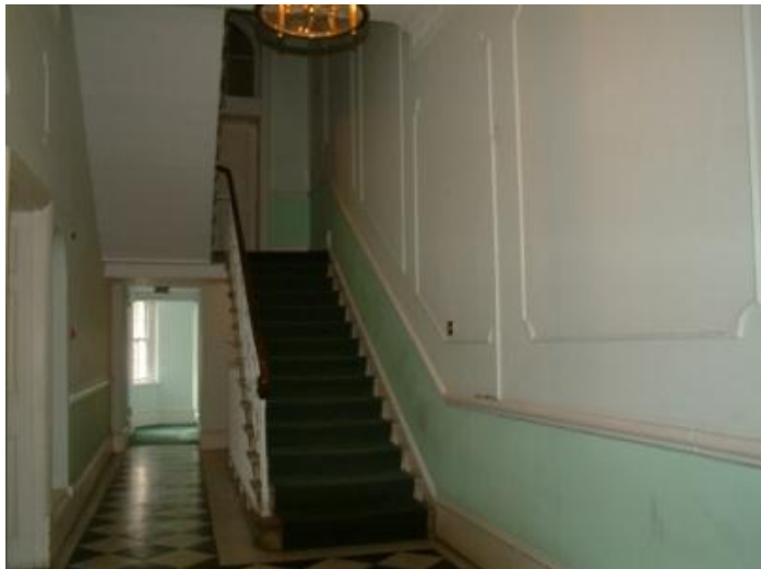
Stone Staircase with S-scroll balusters in 2008 prior to refurbishment
