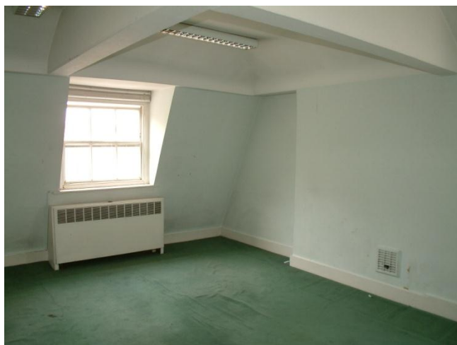
3 rd Floor front room in 2008 prior to refurbishment
