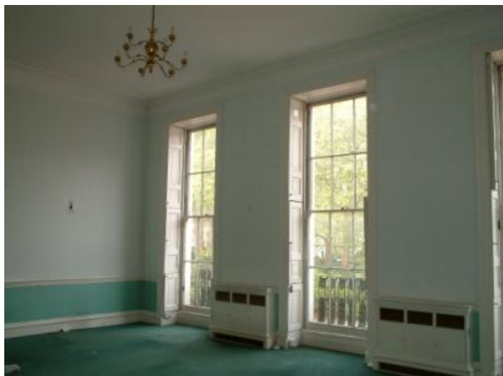
First floor timber sash windows and shuttering in 2008 prior to refurbishment
