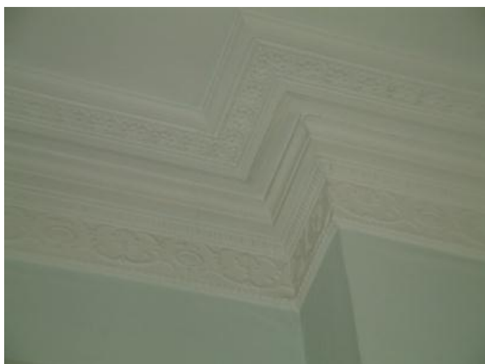
1 st Floor Back Room Cornice in 2008 prior to refurbishment
