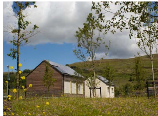
South elevation of the Larch and Lime Passivhaus dwellings
