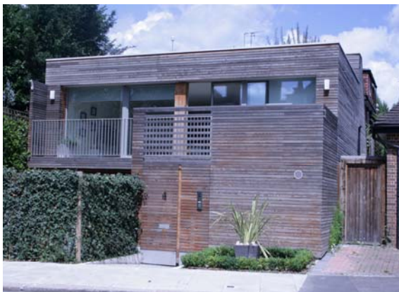
Street View of the Camden Passivhaus
