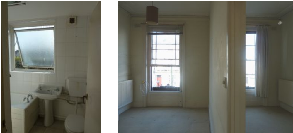
Fig.10 The current bathroom within the rear extension – note the aluminium window to be replaced with a glazed timber door and casement under the retained lintel.
