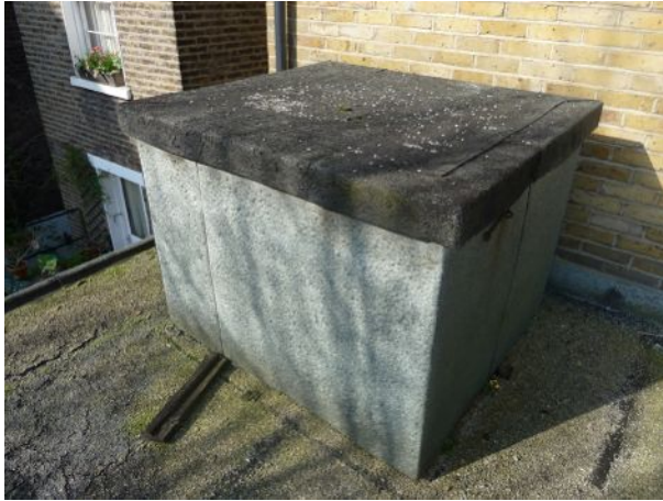
Fig.4 Water tank to be removed
