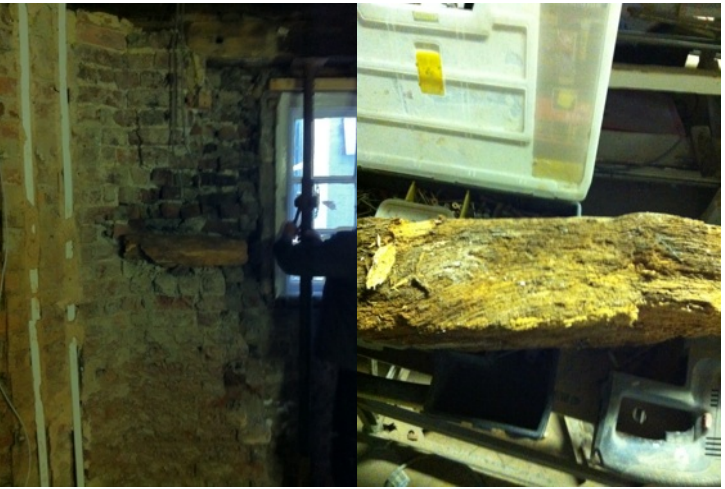
rotten timber removed from wall to rear bay
