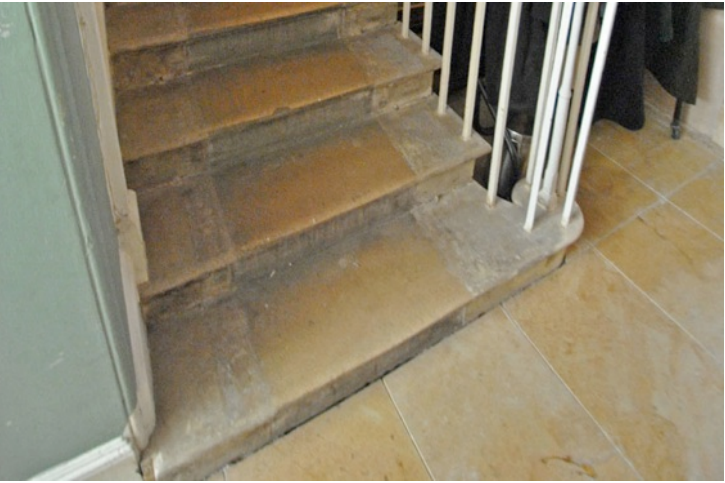
limestone slabs replacing concrete in hallway at base of stairs
