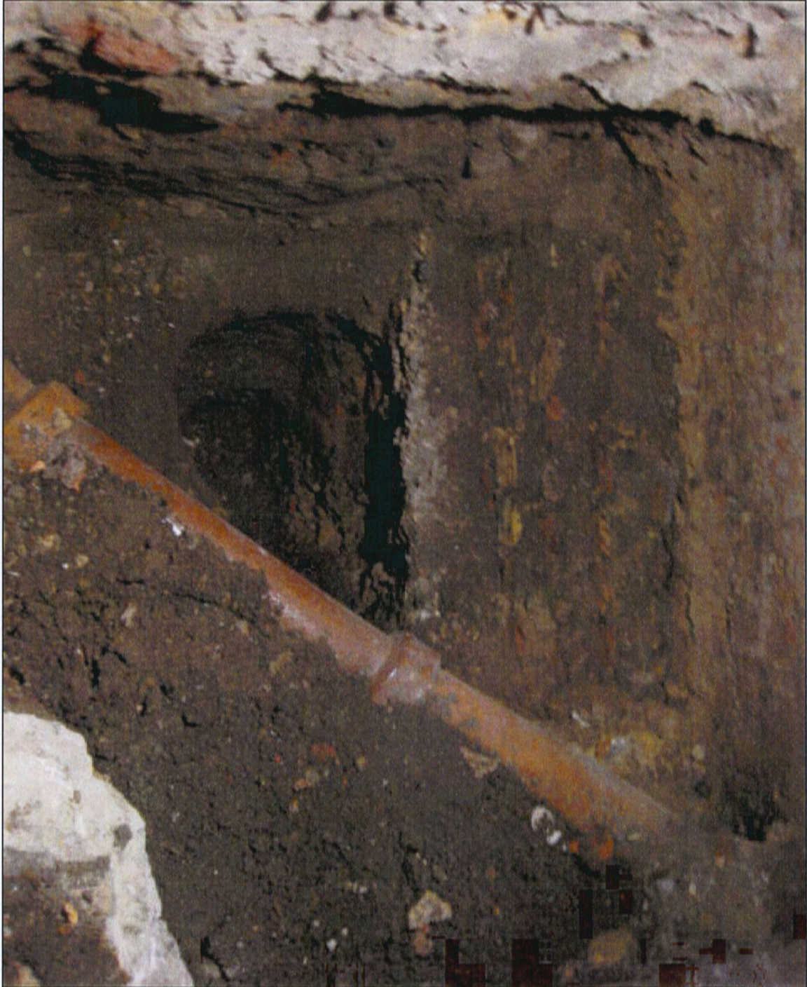
View of the footings encountered in Trial Pit No 12, looking west (19/05/2011)
