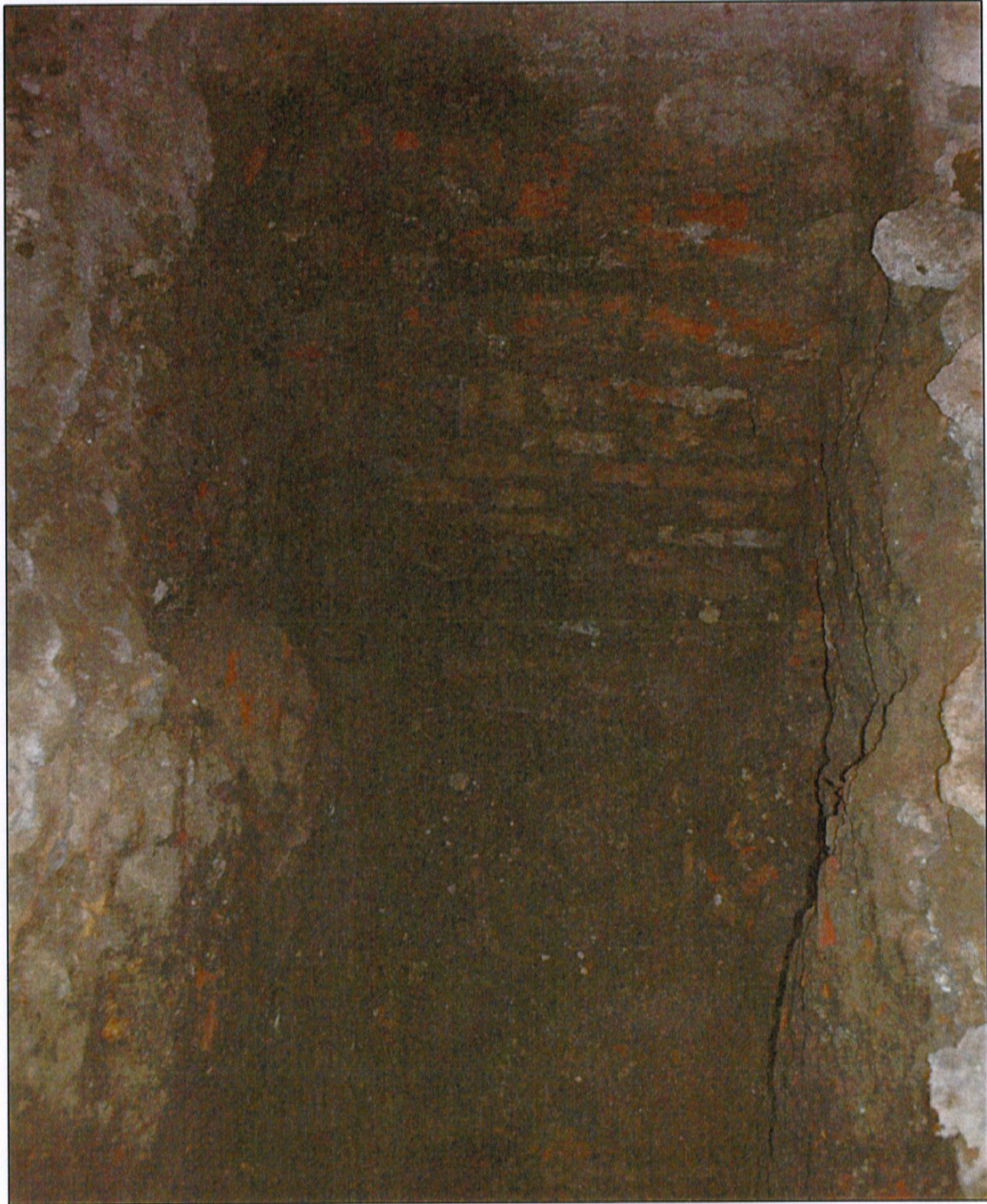
View of the footings in Trial Pit No 9, looking south (20/05/2011)
