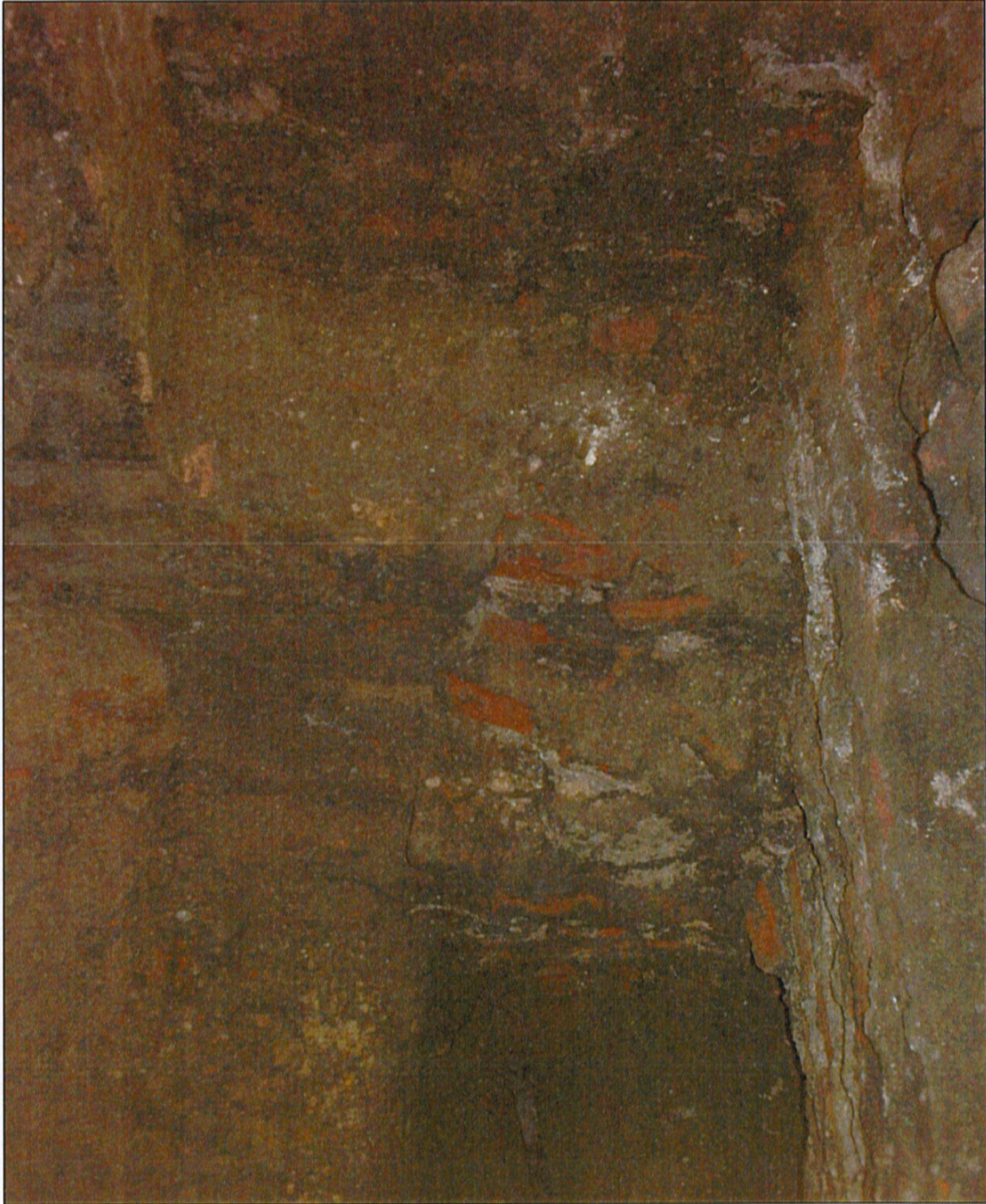
View of the footings encountered in Trial Pit No 8, looking north (20/05/2011)
