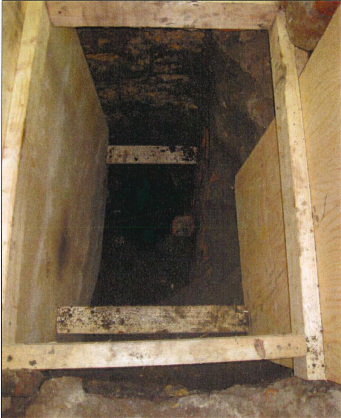
View of the footings in Trial Pit No 3, looking north (19/05/2011)
