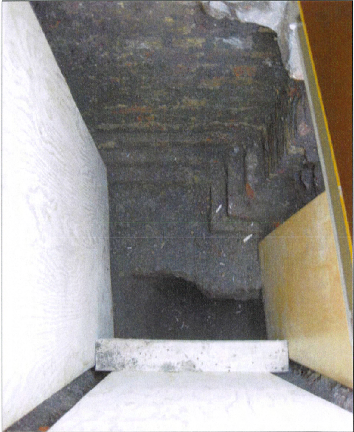
View of the footings encountered in Trial Pit No 1, looking east (19/05/2011)
