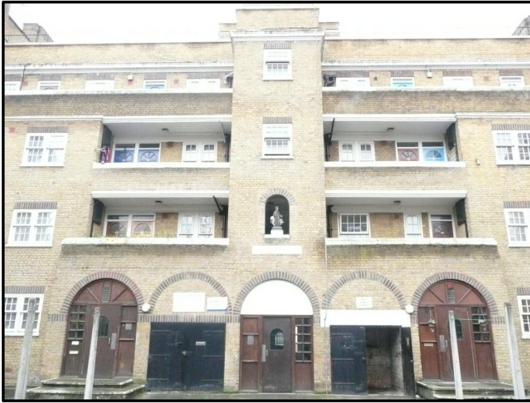
Fig. 1: Front Elevation St Anthony's Flats
