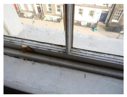
Windows to Gower Street showing original vertical sliding shutters now removed and modern sash replacement window.
