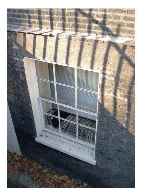
**APPENDIX K** Basement Gower Street- 15mm glazing bars with slight moulding.
