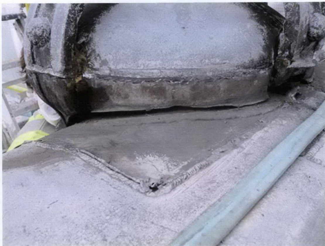
Figure 20. Removal of Crown
