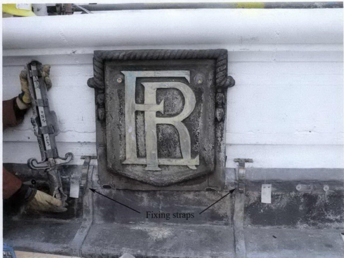
Figure 6. Sword armature and lower fixing straps
