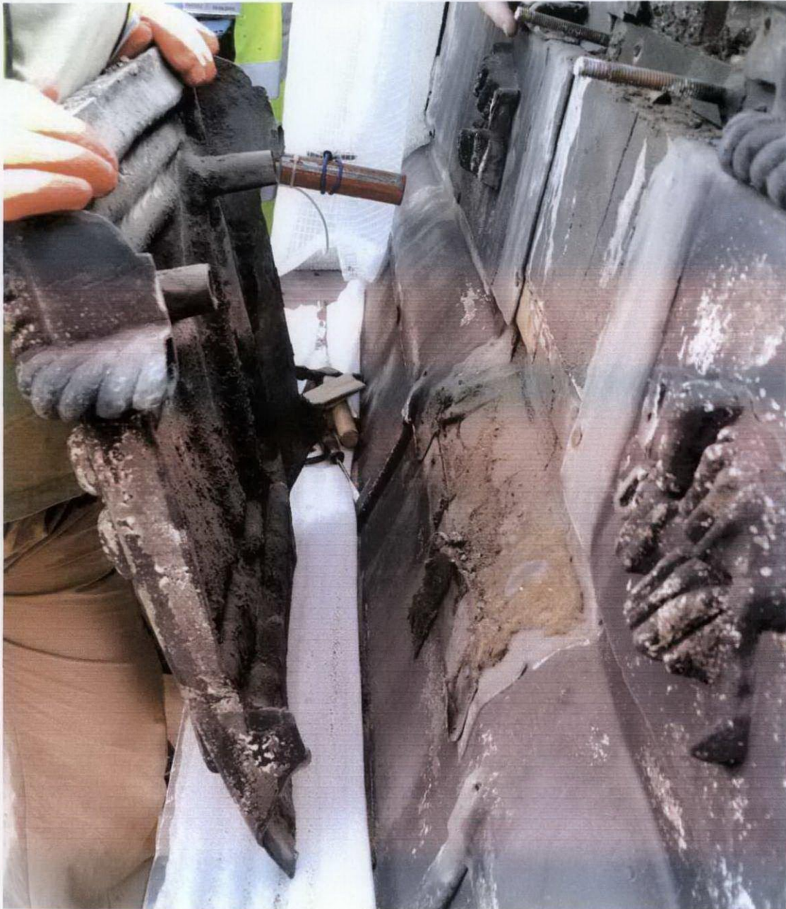
Figure 4. Shield during removal
