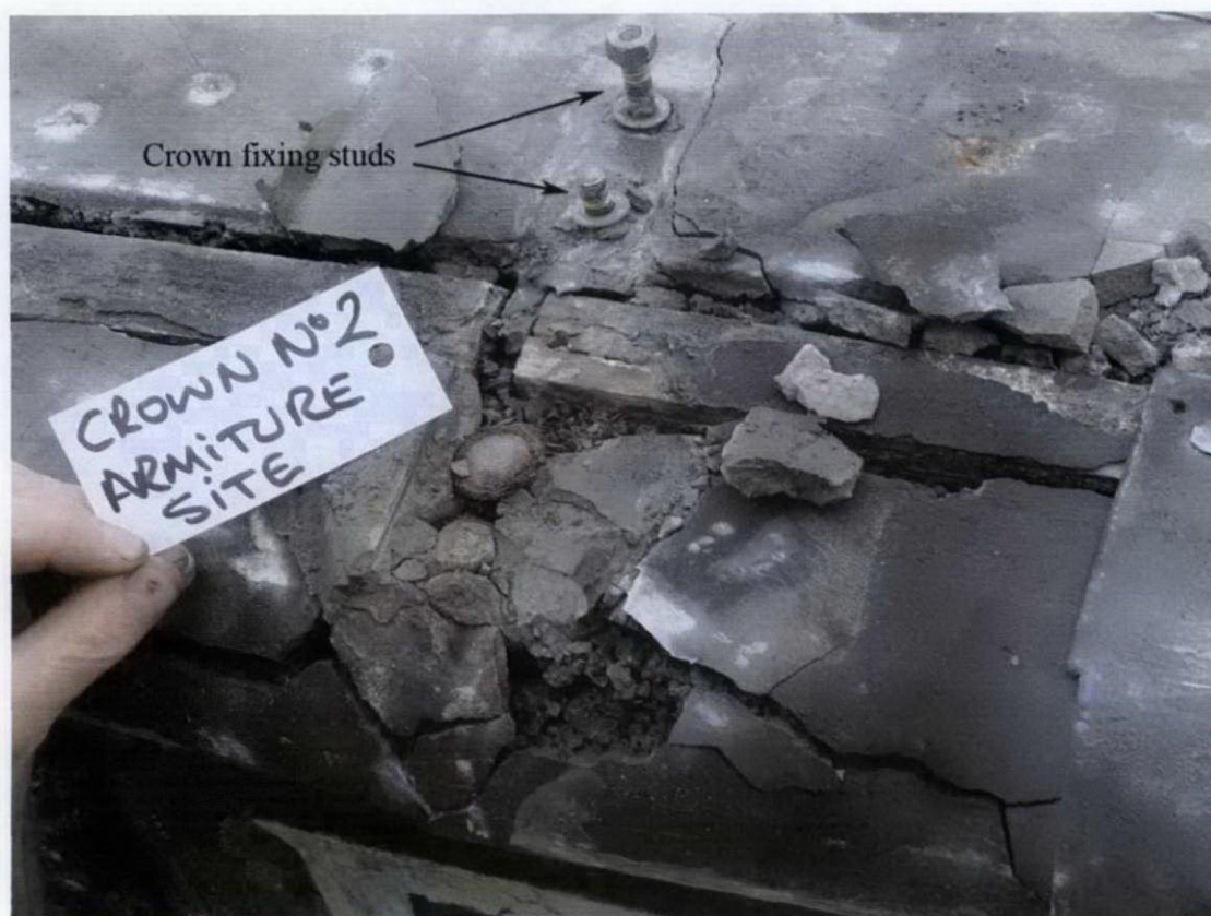
Figure 23. Top of parapet after removal
