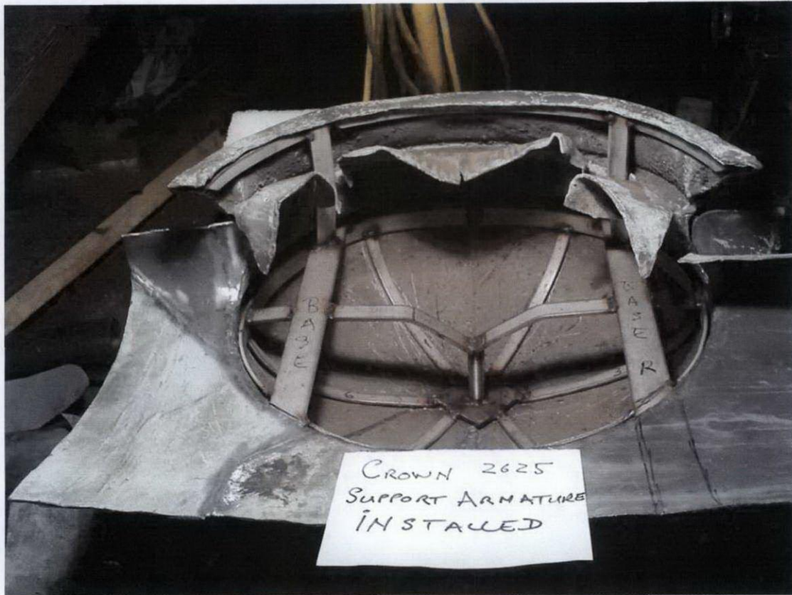
Figure 26. Installation of new support armature
