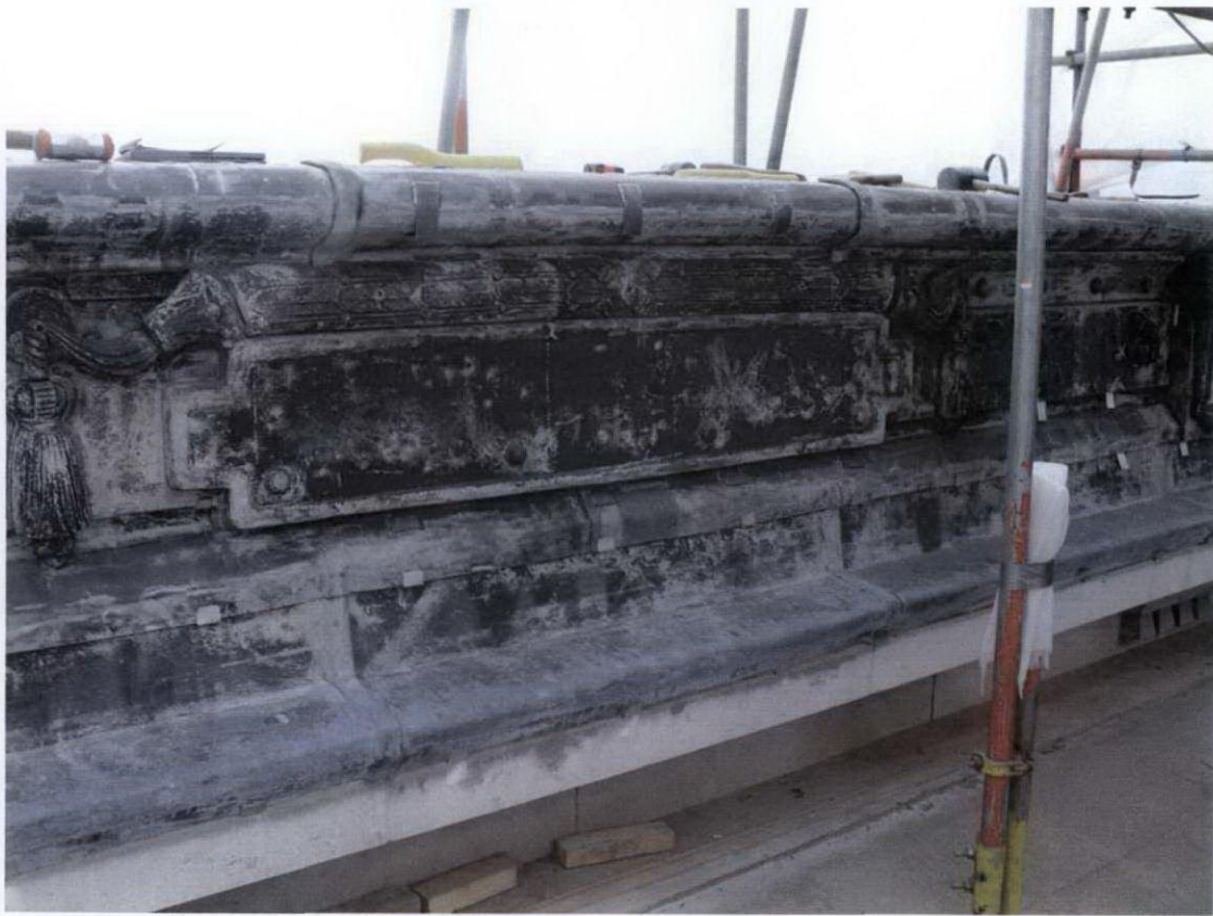
Figure 14. Swags in place
