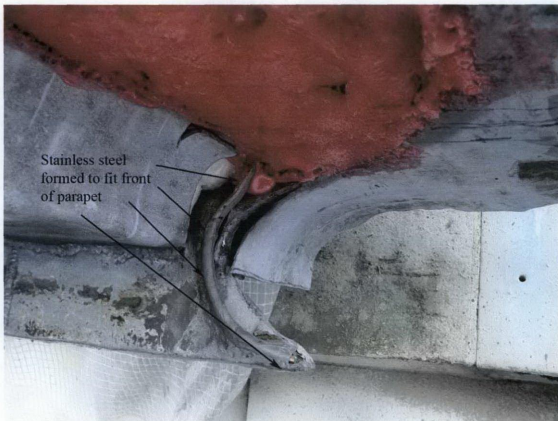
Figure 29. Underneath front of Crown, showing armature detail
