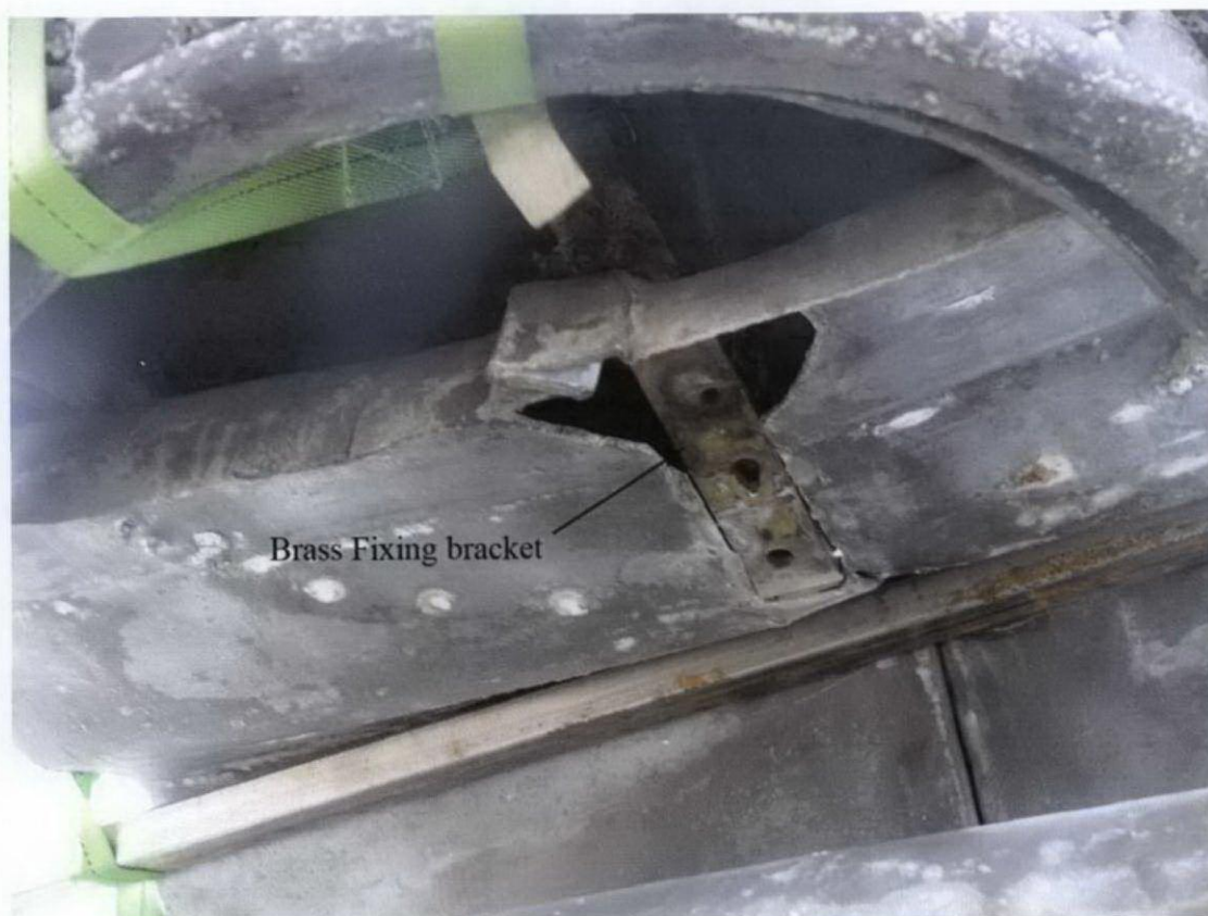
Figure 22. Underneath removed Crown
