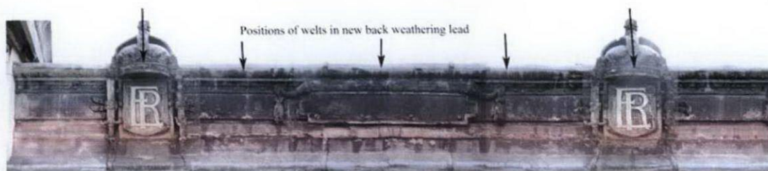
Figure 3. Position of welts in new lead at back
