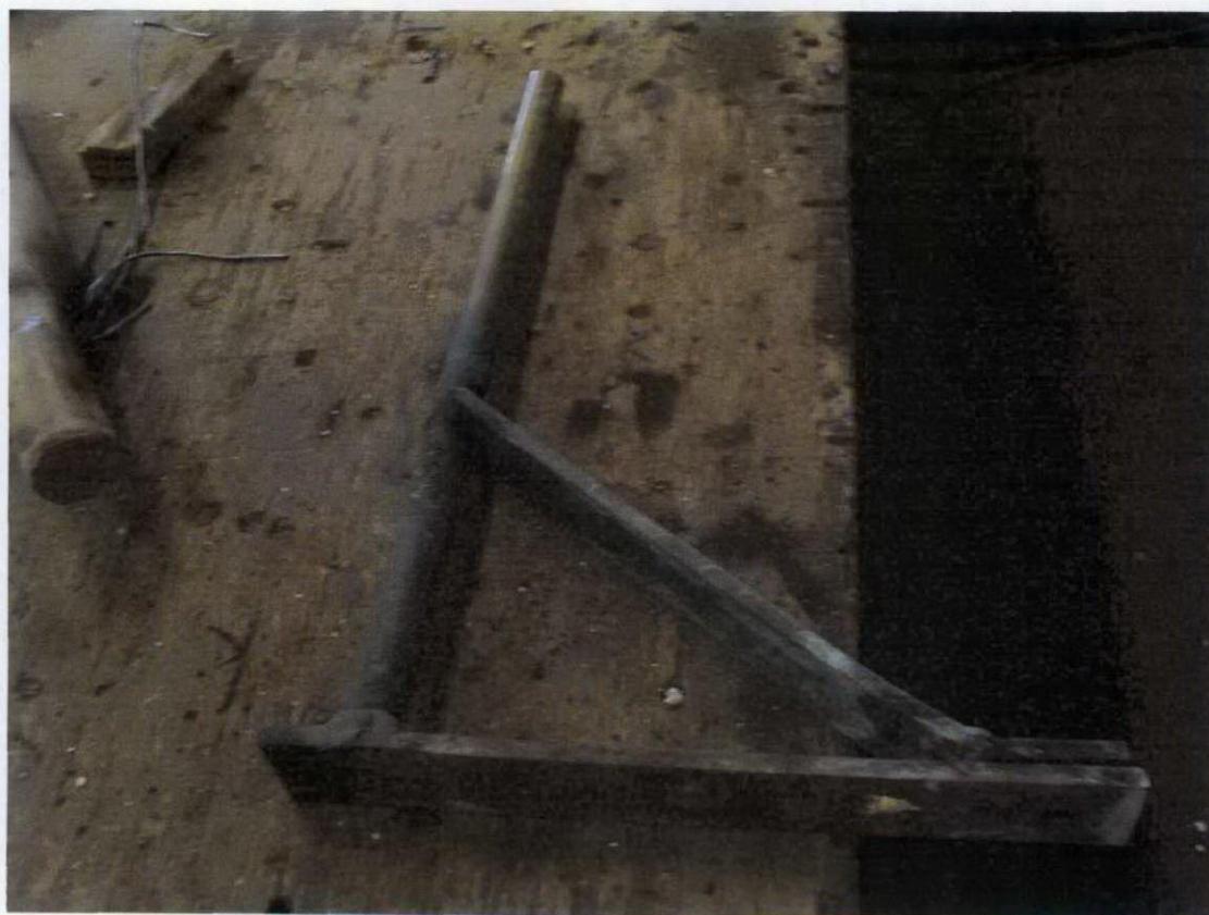
Figure 25. Crown fixing bracket removed
