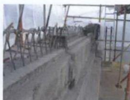
Before Sandblasting 30-7-C
