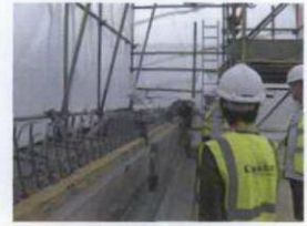
BM North Facade 001.jpg
