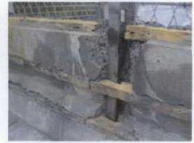
BM North Facade 006.jpg
