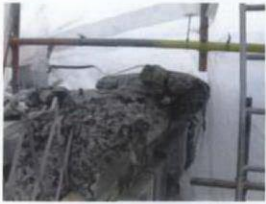
BM North Facade 002.jpg
