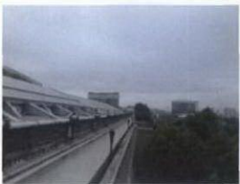
BM North Facade 007.jpg
