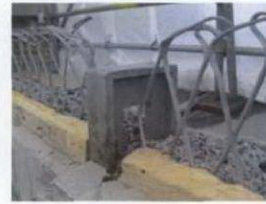
BM North Facade 005.jpg
