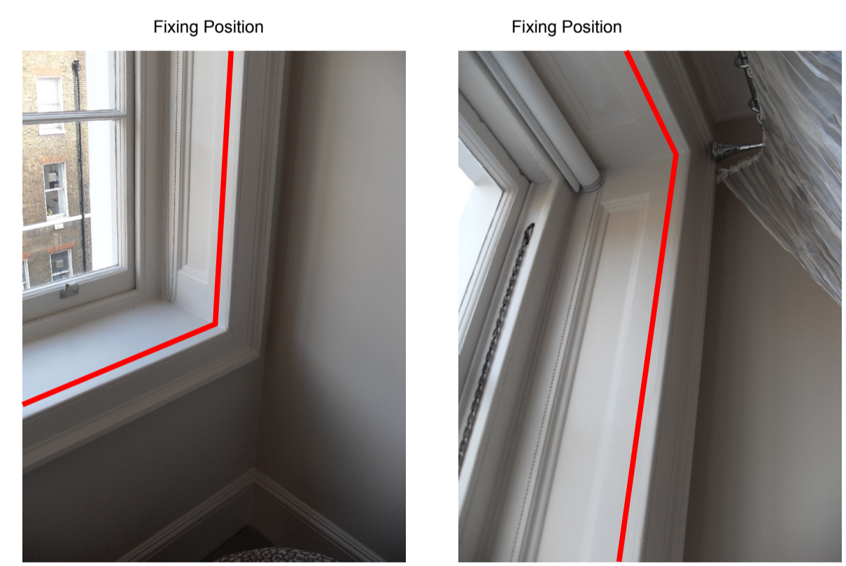
EXISTING WINDOW PHOTOGRAPHS
