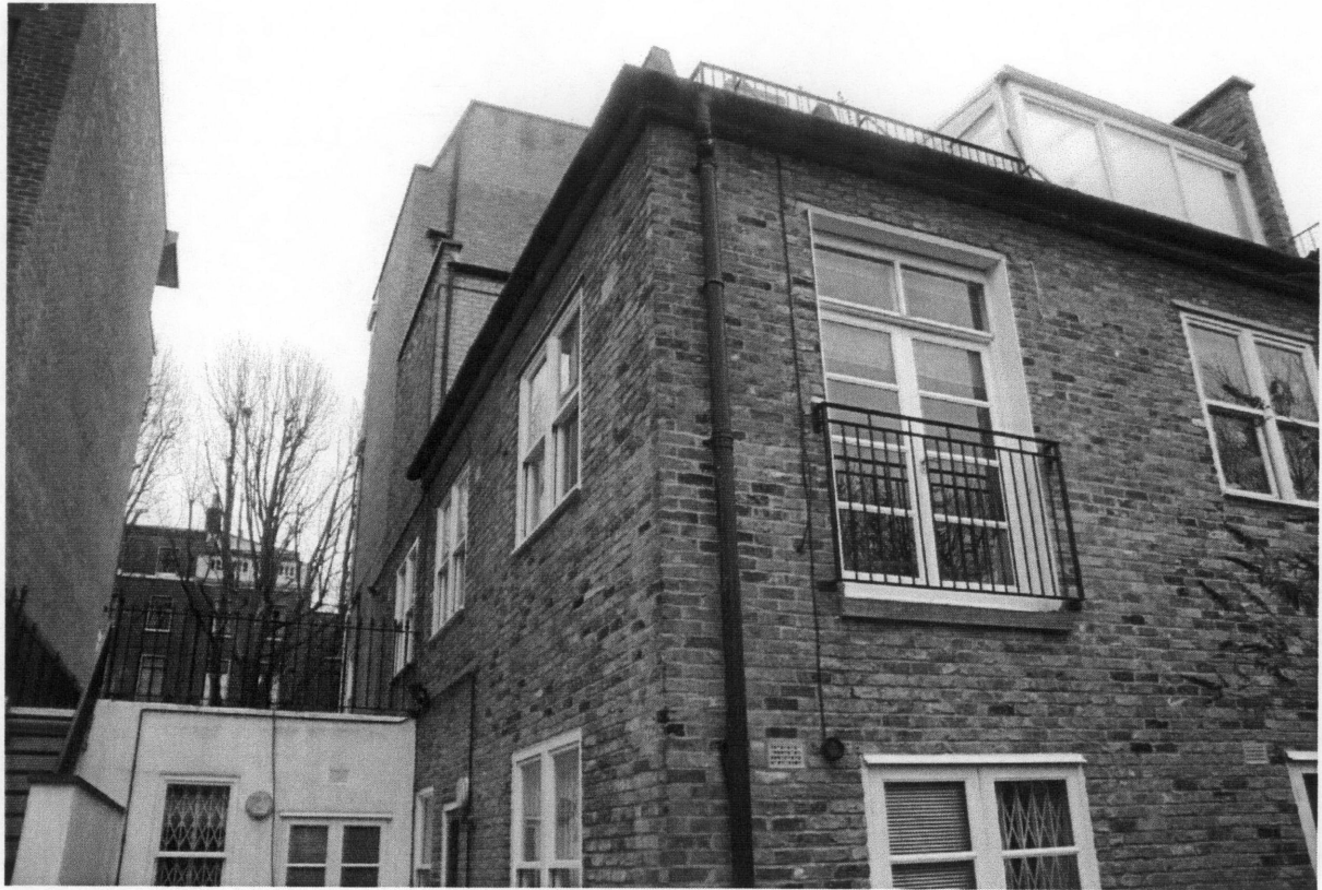
3) Upper part of rear elevation.
