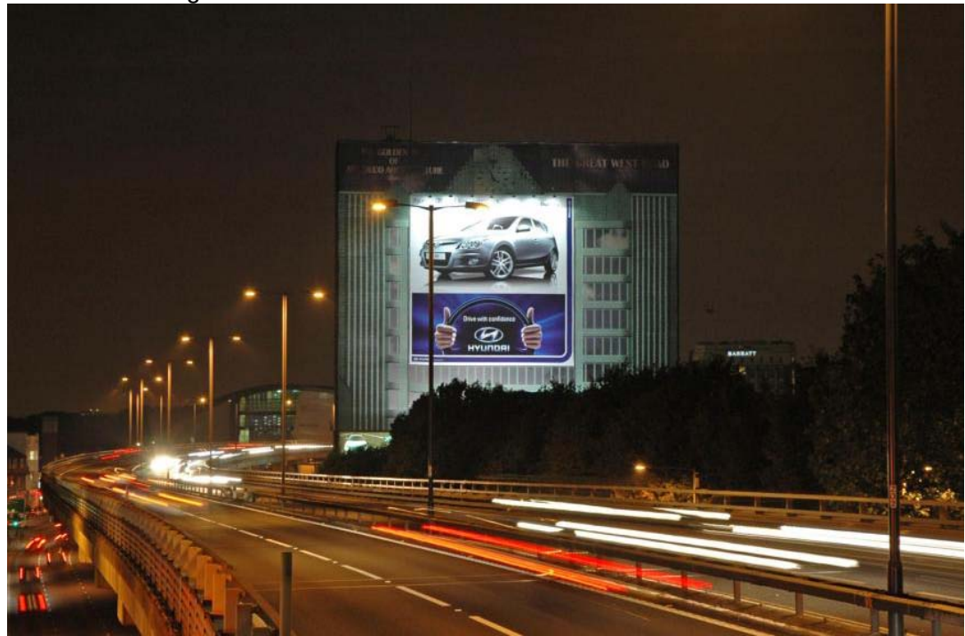
Alfa Laval Building M4 Elevated section London
