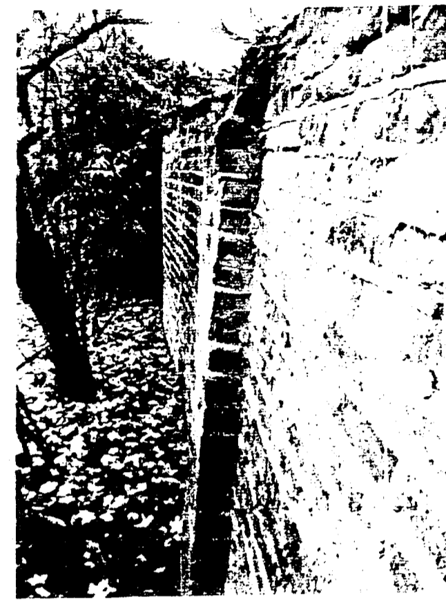
Lean in wall towards rear of garden
