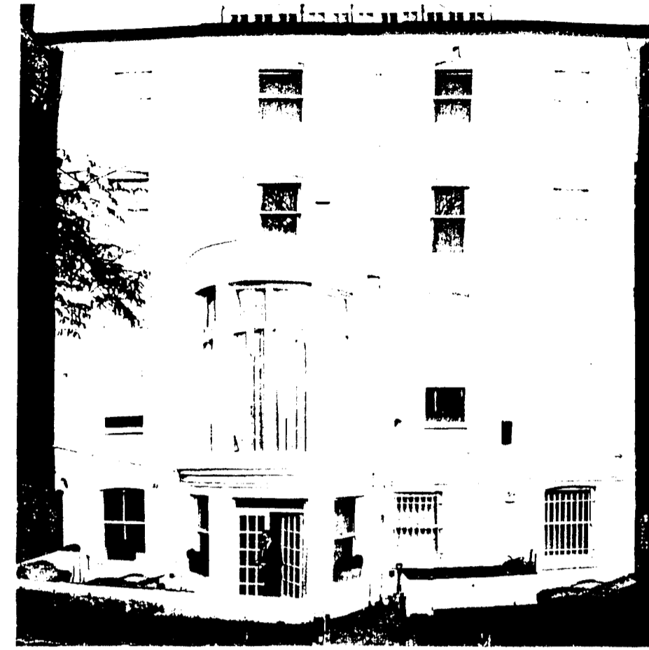
existing view of rear elevation
