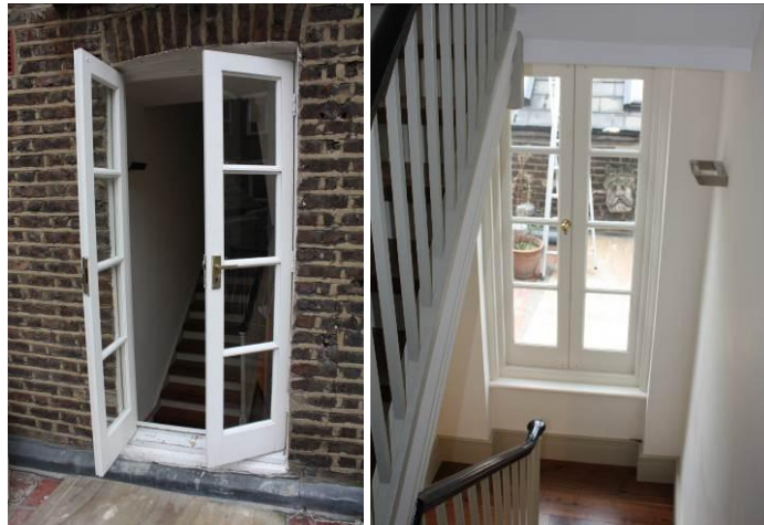
Photograph 3 and 4 - French door external and internal (dated 16.02.2012)
