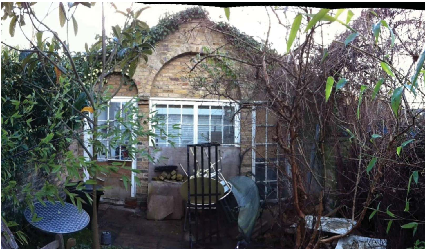
D. View of garden elevation of garage
