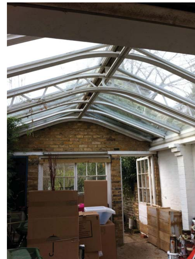
E. Interior view of garage
