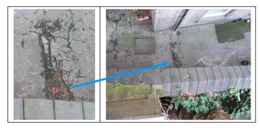
In addition to this the neighbouring footpath has suffered direct damage from tree roots as shown in the photograph opposite which could form a trip hazard.
