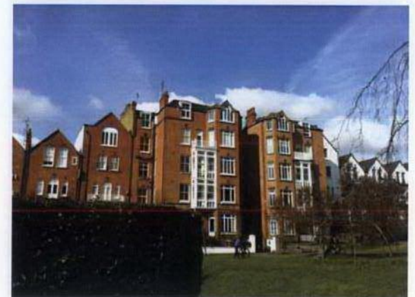
5 37 Canfield Gardens viewed from rear gardens showing adjacent properties
