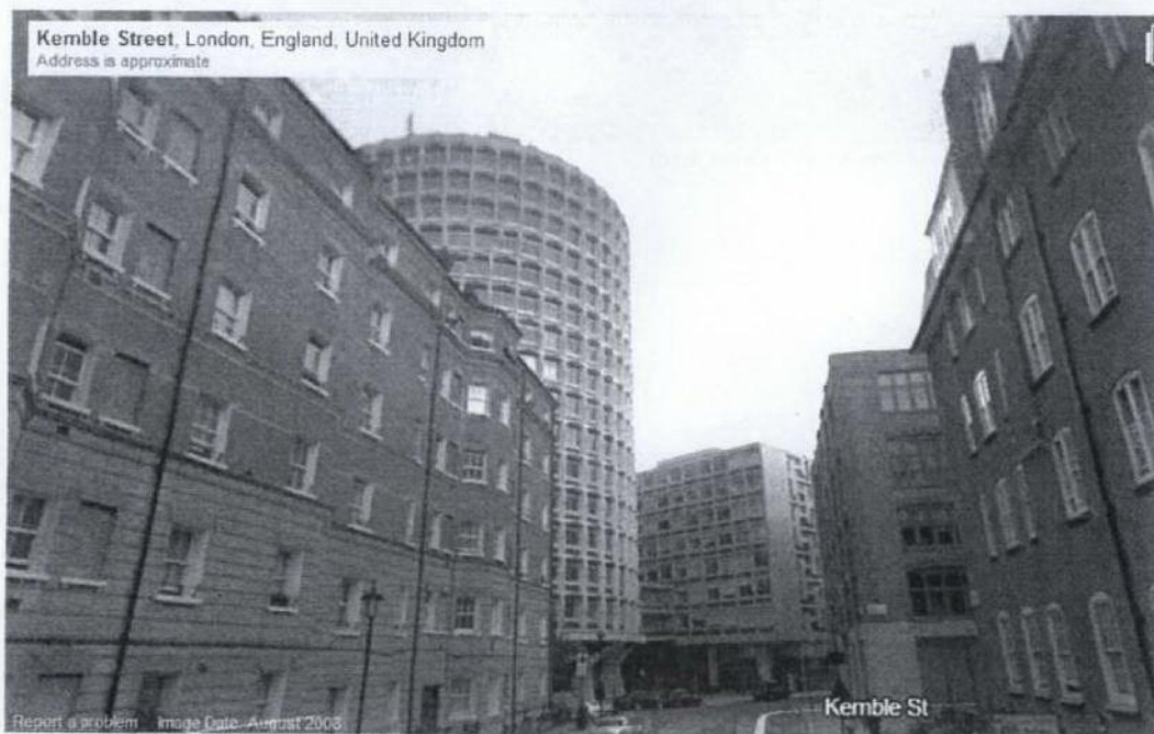
Figure 1 - View of One Kemble Street (Tallest Building)
