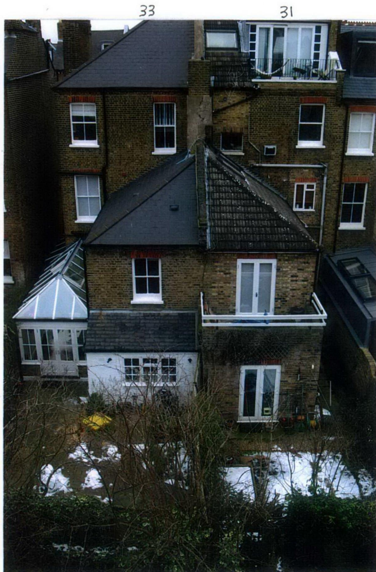
VIEW OF EXISTING REAR ELEVATIONS
