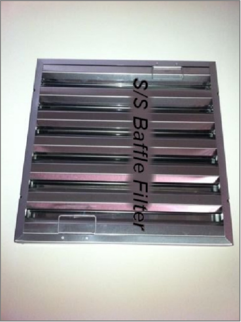
EXISTING BAFFLE GREASE FILTERS WITHIN KITCHEN CANOPY
