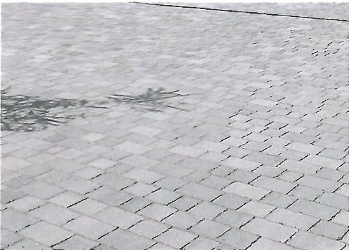
Marshall Tegula Pennant Grey - Paving to Access Way Colour: Grey Finish: Rumbled
