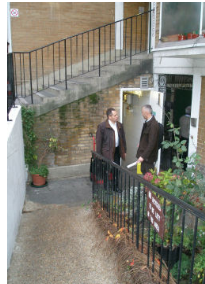
Existing ramp to lower ground floor level does not comply with Building regulations.
