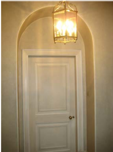
4 | PHOTOGRAPH TYPICAL EXISTING DOOR 30 | NTS
