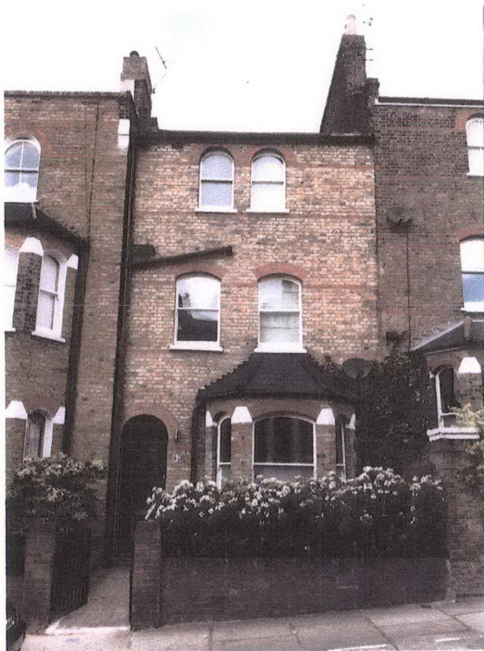
PHOTOGRAPH OF FRONT ELEVATION ( CHETWYND RD )
