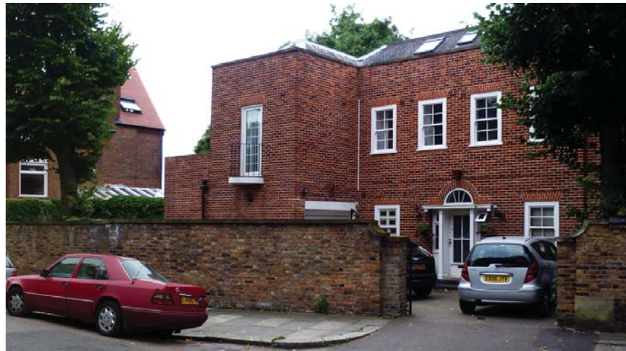
VIEW 1 - No.6 NUTLEY TERRACE, VIEW FROM NUTLEY TERRACE
