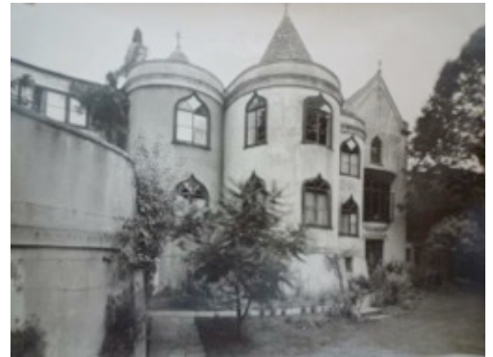
Dividing wall built sometime between 1916-1930
