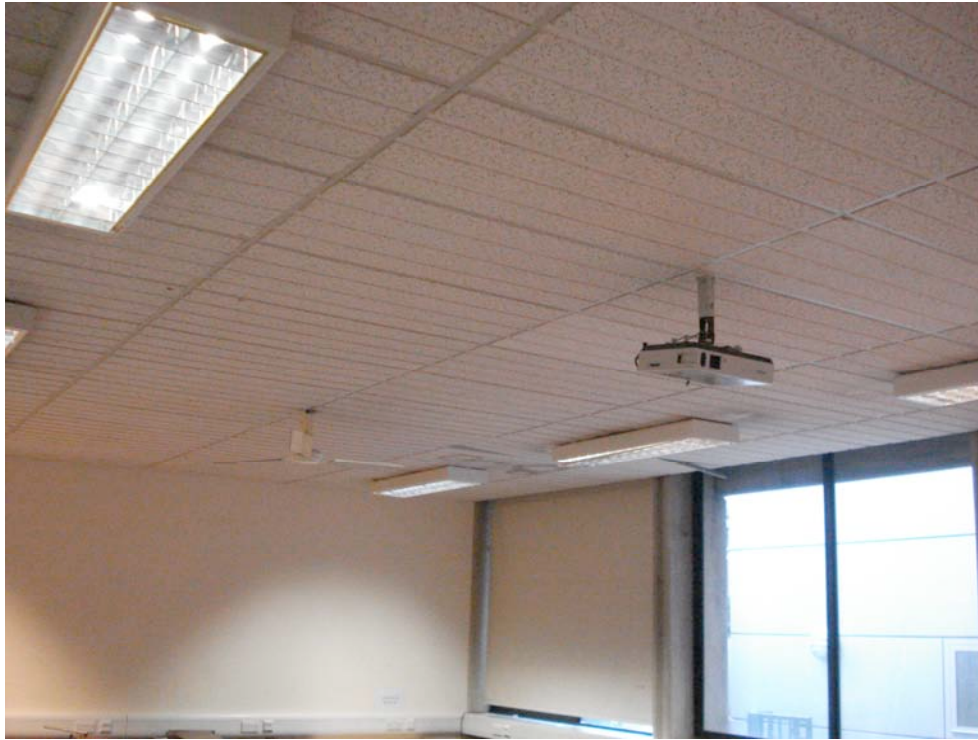
Photograph 03 – Suspended ceiling in L67 to be replaced for plaster boarded ceiling.
