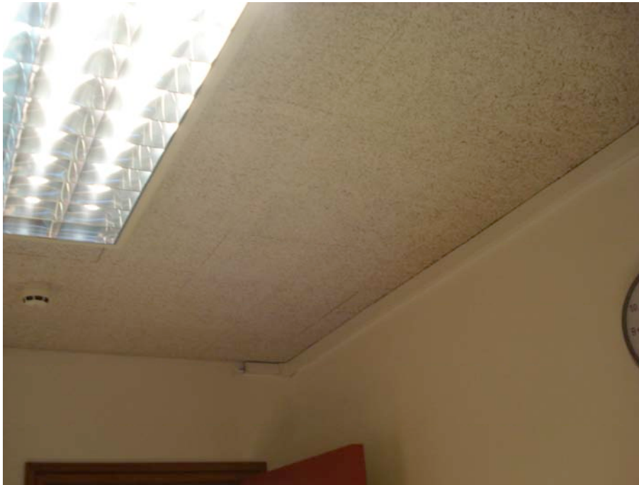
Photograph 02 – Existing suspended ceiling to be replaced with new plasterboard ceiling.
