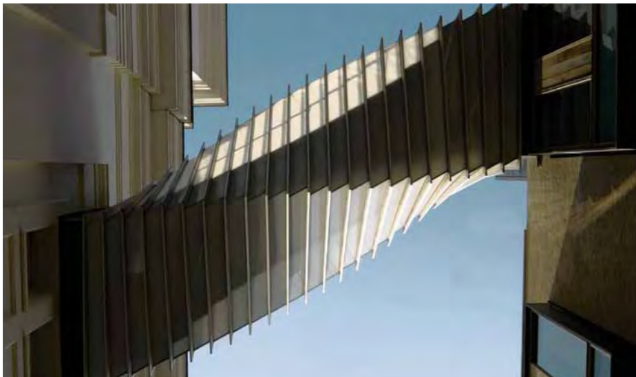
Wilkinson Eyre's bridge link to the grade 1 listed Royal Ballet School, London
