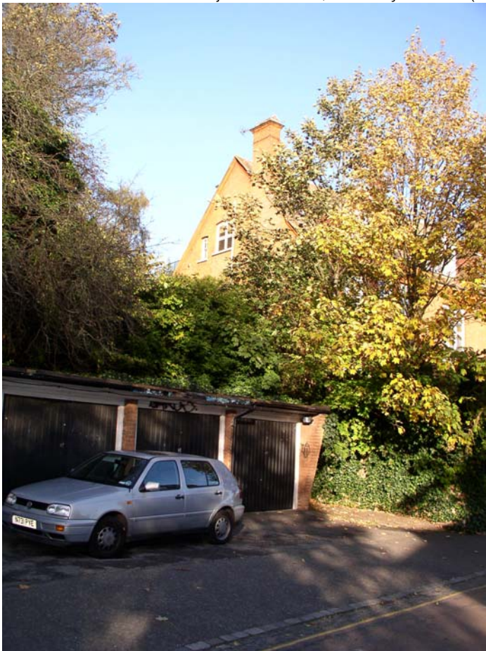
Photo No. 4 – View of garages 3-6 and 3 Nutley Terrace
