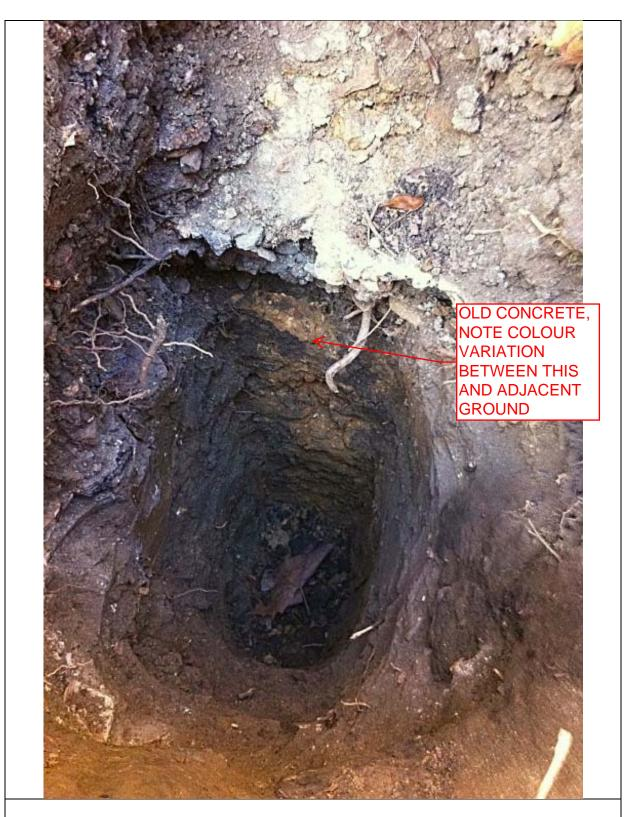
TRIAL PIT DUG AT RADLETT HOUSE ADJACENT TO PRIMROSE HILL BOUNDARY WALL TO INSPECT FOOTINGS DETAIL  ${\bf 13}^{\text{TH}}$  DECEMBER 2011.
