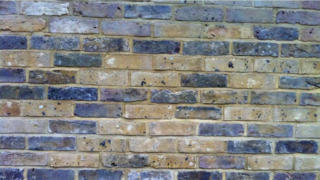
RECLAIMED YELLOW LONDON STOCKS POINTING TO MATCH EXISTING DR NO.: 1001-PH-0006
