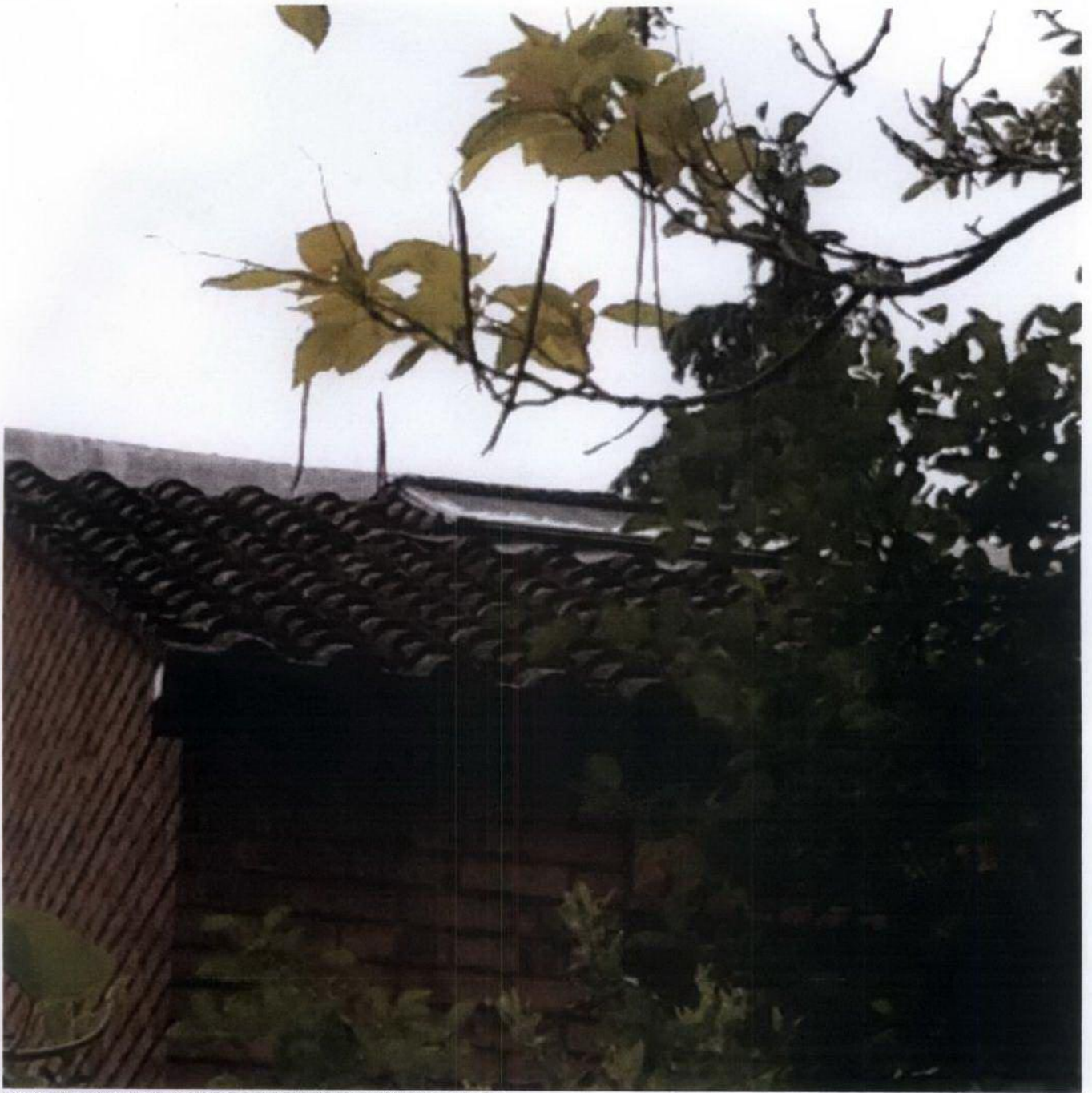
Identical rooflight in the same position installed at 34 West Hill Park
