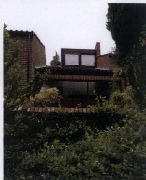
View of the rear elevation of 35 West Hill Park
