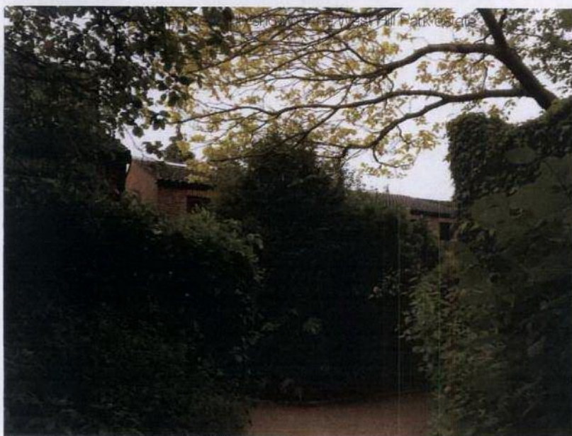
View of the rear elevation of 35 West Hill Park
