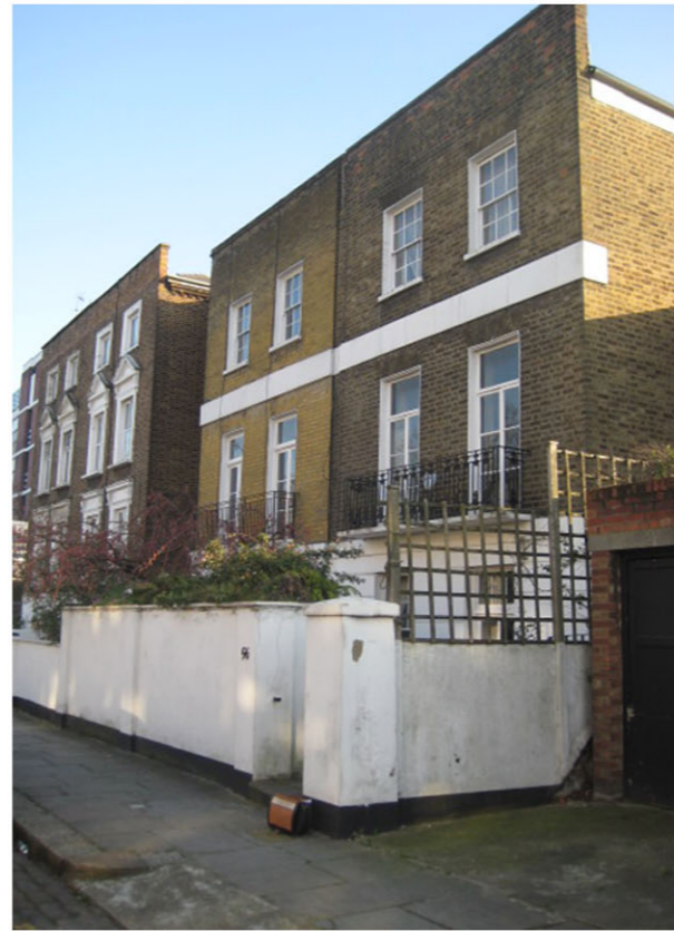
56 Rochester Road with Garages to the right
