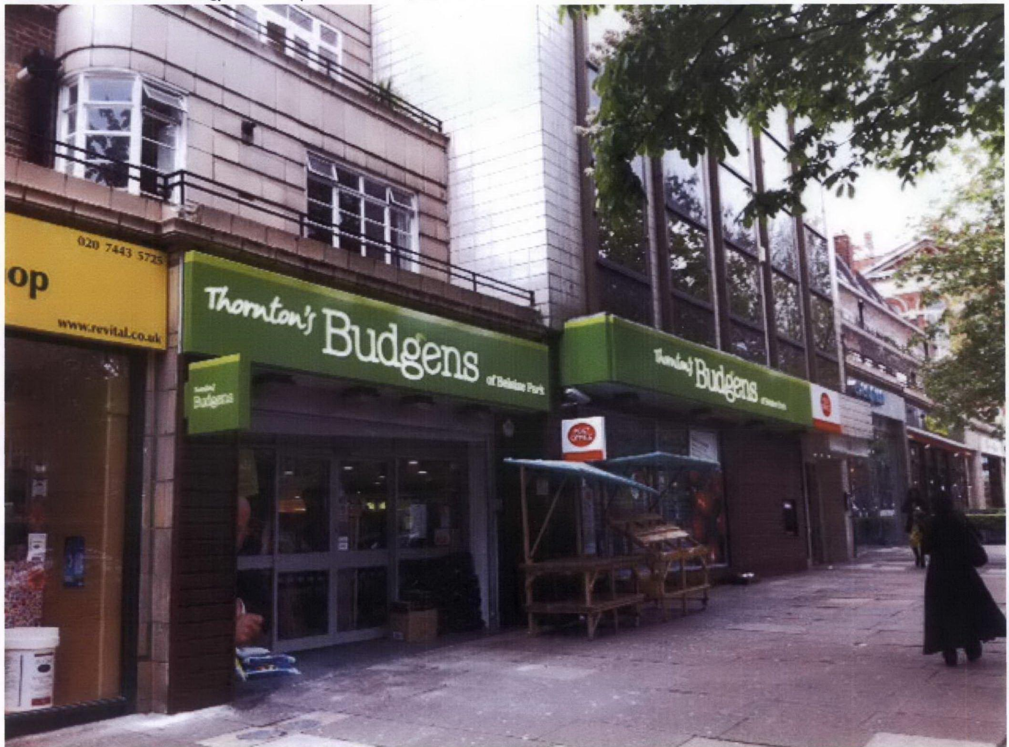
CLADDING COMPLETION PICTURE
