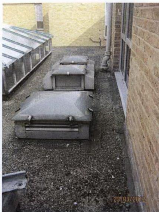
Photo 2 – Kitchen roof: Existing rooflights to be removed
