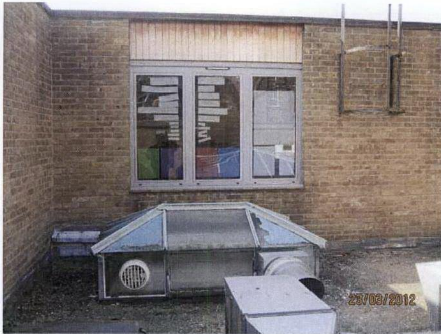
Photo 3 – Kitchen roof: Existing rooflights to be removed
