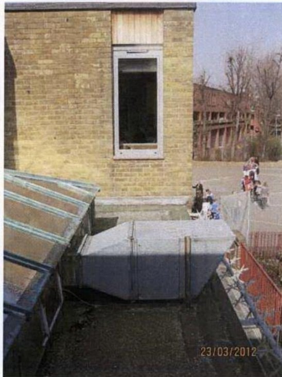
Photo 5 – Kitchen roof edge to be provided with guarding
