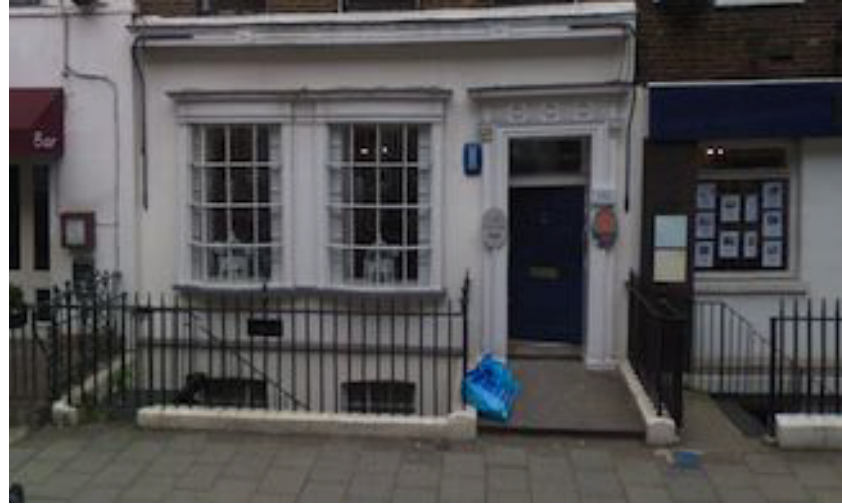
FRONT RAILINGS & LIGHTWELL AT 72 CHARLOTTE STREET
