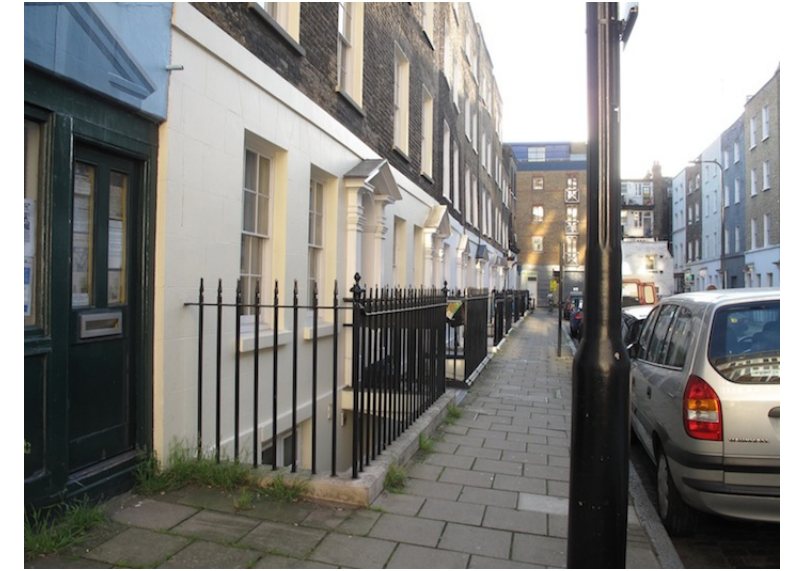
VIEW OF FRONT LIGHTWELLS AND RAILINGS AT GODGE PLACE
