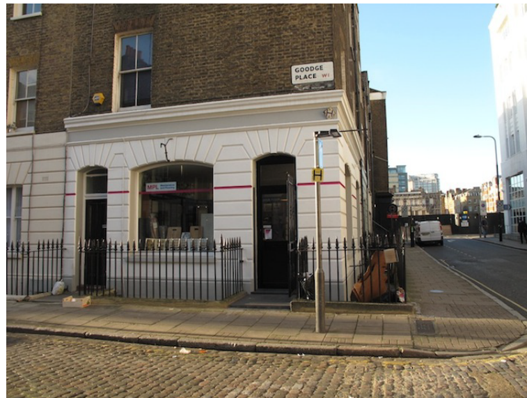
TOTTENHAM STREET & GODGE PLACE SHOWING A BASEMENT LIGHTWELL WITH RAILINGS WRAPPING AROUND THE CORNER OF THE BUILDING
