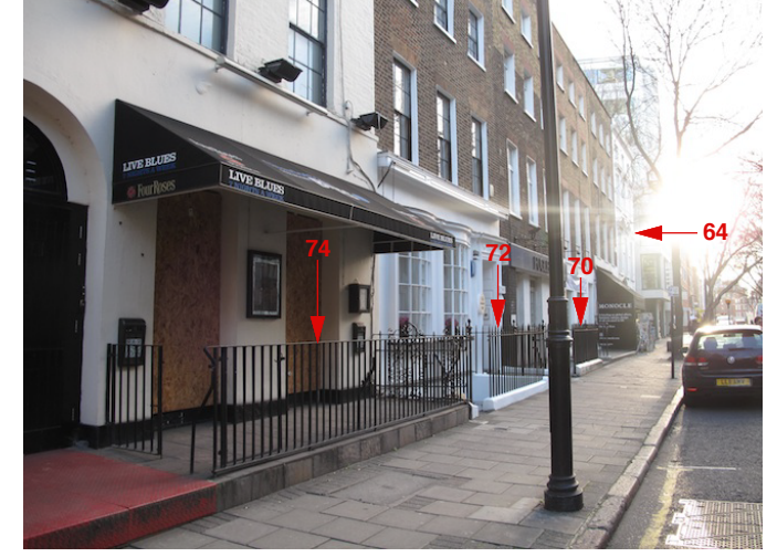
VIEW LOOKING DOWN CHARLOTTE STREET SHOWING FRONT RAILINGS AT NOS. 74, 72, 70
