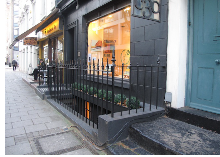
FRONT RAILINGS & LIGHTWELL AT 30 TOTTENHAM STREET
