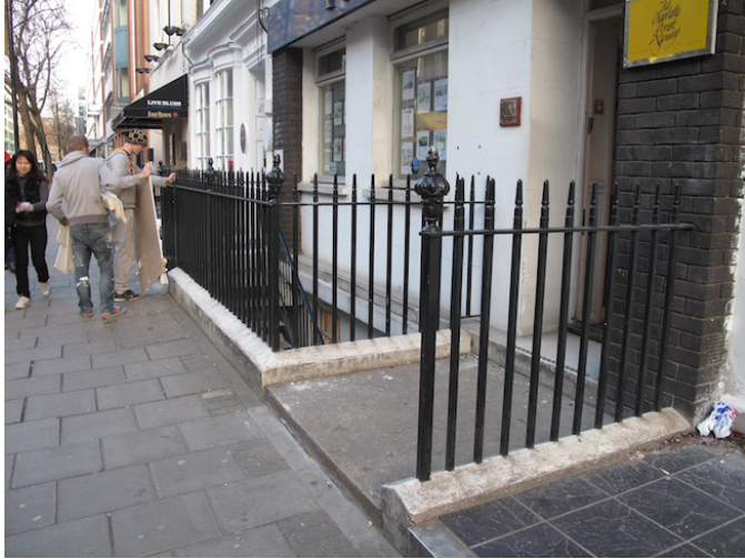
FRONT RAILINGS & LIGHTWELL AT 70 CHARLOTTE STREET
