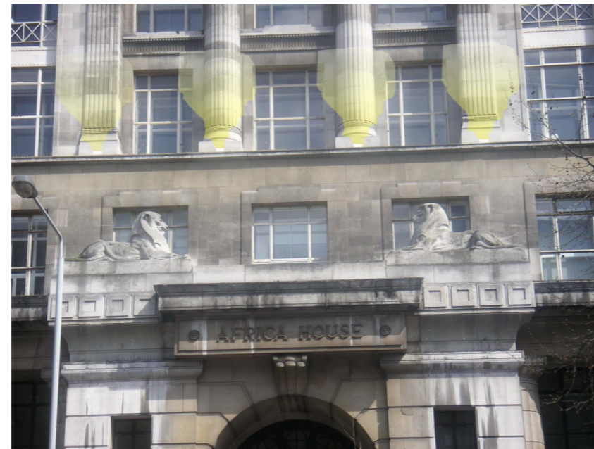
C Photomontage showing AWA 15003 halide luminaires lighting 4 main columns - 3rd floor
