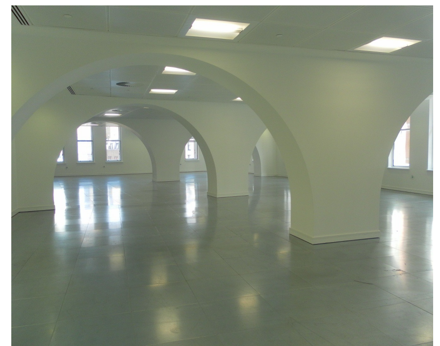
Figure 5: A view of the same space today, illustrating the extent to which historic features have now been concealed by plasterboard, raised floors and suspended ceilings.
