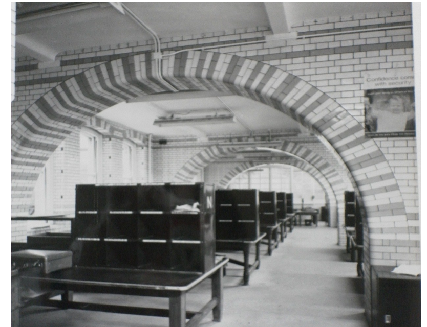
Figure 4: A view of the interiors of the former 'Ridler's Hotel' Block, in the south-east section of 2 Waterhouse Square, as they appeared in use by the Prudential in 1968. Glazed brick arches dominate here.
