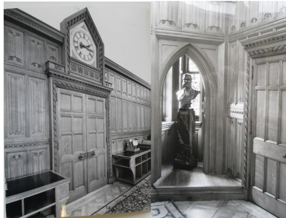
Figure 6: Internal views of panelled, directorial rooms within the former Prudential Offices. The 'linenfold' panelling found in these rooms matches that which Waterhouse designed for the original building's Boardroom in the late 1870s, and which can now be found in the former Director's Rest Room (figure 7).
