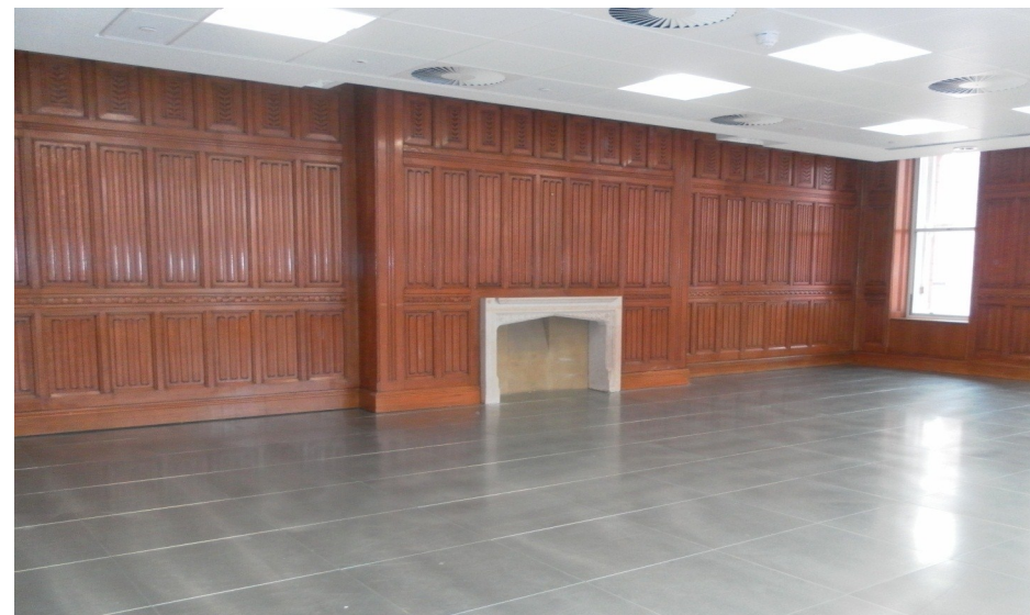
Figure 7: The former Director's Rest Room as it appears today. The appearance of its linenfold panelling and simple, stone Neo-Gothic fireplace has been harmed to an extent by the introduction of later office features, such as suspended ceilings.
