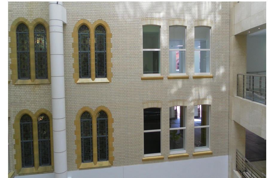
Figure 9: A view of the glazed brick, formerly open, lightwell, within 2 Waterhouse Square. The elaborate, stained glass Gothic windows to the left of this image relate to one of the staircases, to which no works are proposed.
