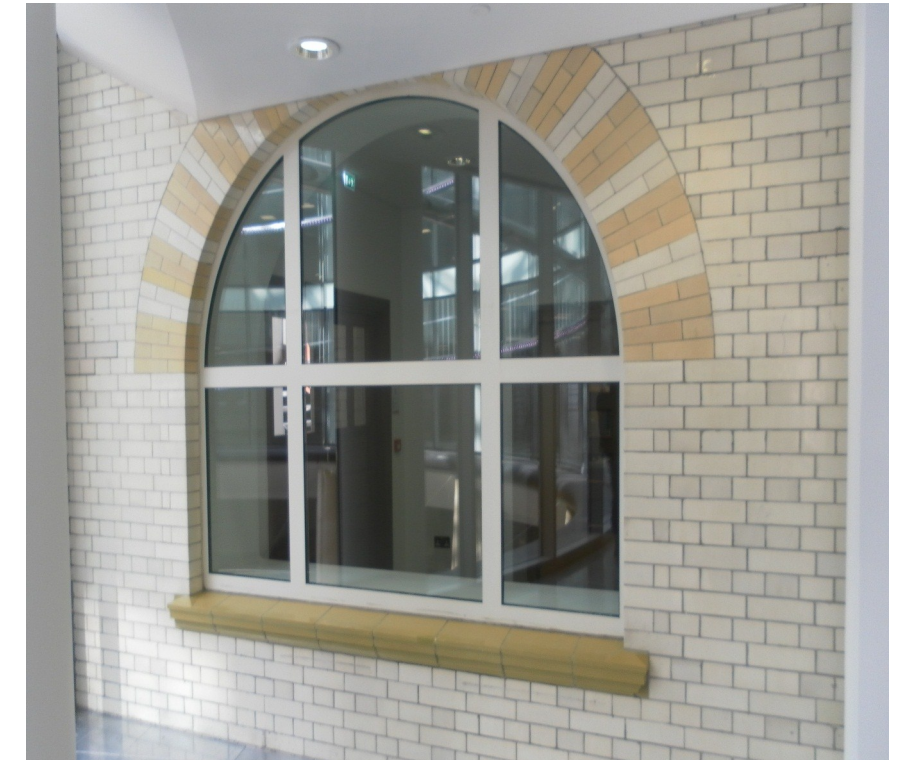
Figure 8: An example of some of the late-Victorian glazed brick that remains exposed within 2 Waterhouse Square.
