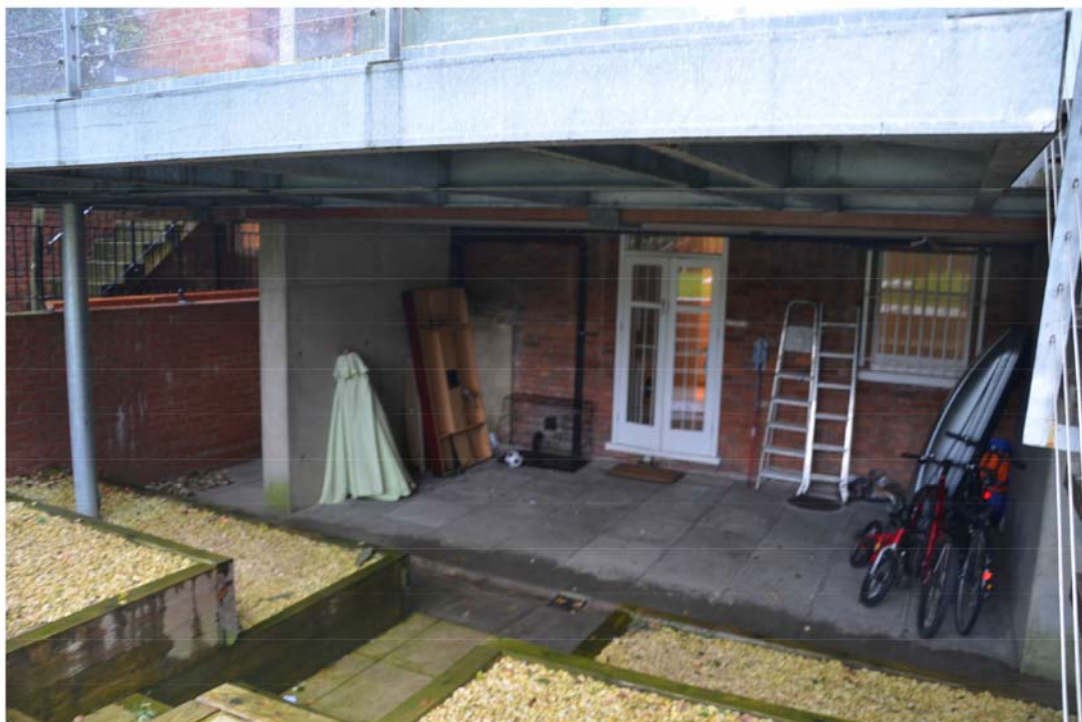
Photograph 5 : Void beneath metal decking, reducing natural light to the lower ground floor
