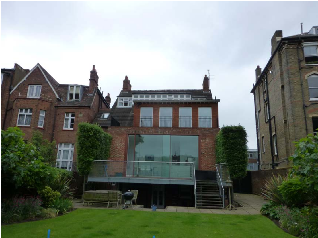
Photograph 3 : Rear garden elevation showing the existing ground floor and first floor extensions and metal decking.
