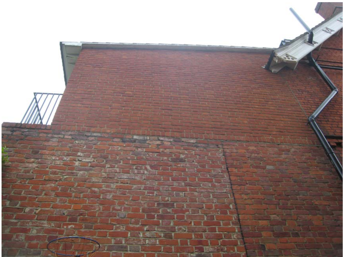
Photograph 8 : Existing overhanging eaves of the shallow pitched roof to modern 1st floor extension
