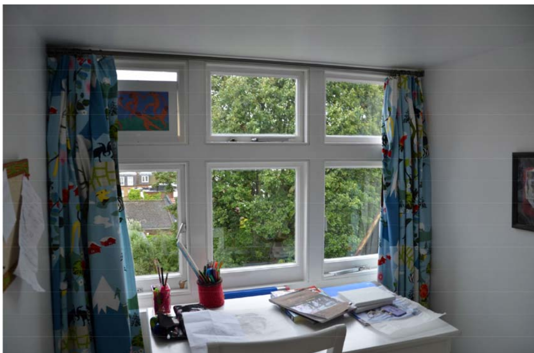
Photograph 6 : Obstructive thick window frames to existing dormer windows at second floor level
